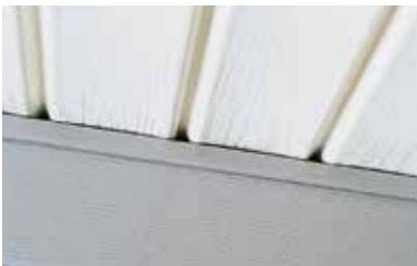
Ordinary soffit lacks stiffness, so it tends to cup when installed.
