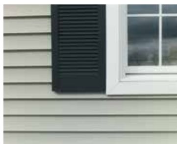
3-1/2" insulated lineal window trim (5" also available)
